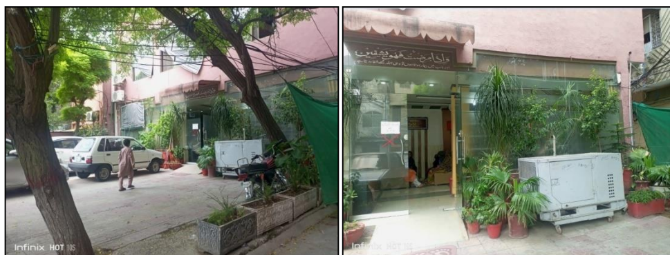
Figure 07 View of the main entrance and parking
