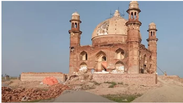
Figure 25 : Work in progress at Dome
