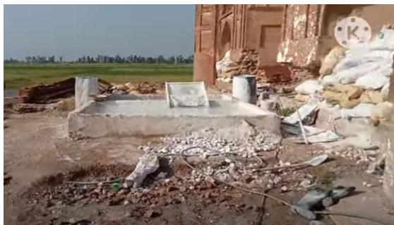
Figure 27: Lime mortar preparation at site
