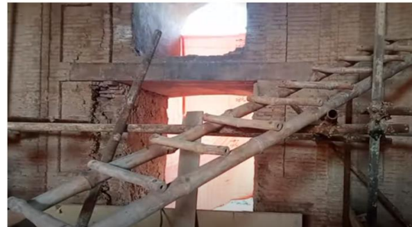
Figure 28: Formwork at Internal side
