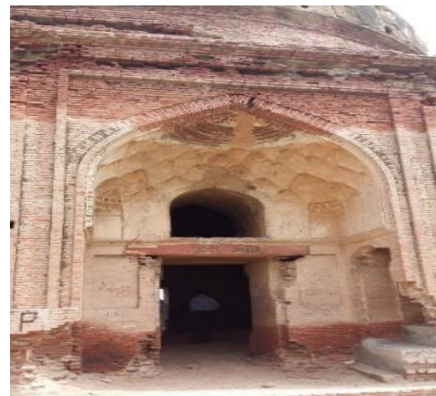
Figure 24: Poor Conservation Technique
