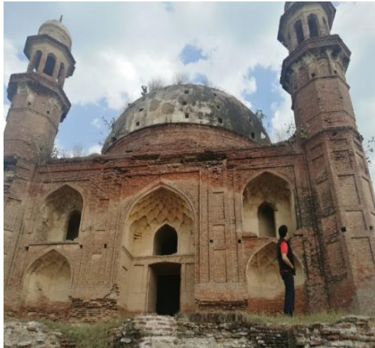
Figure 14: Façade of the tomb showing Climatic effects
