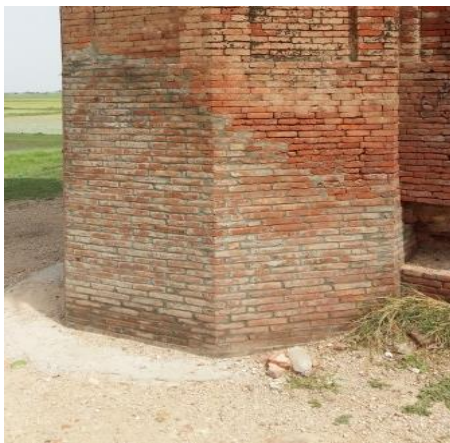
Figure 23 : Repair with cement
