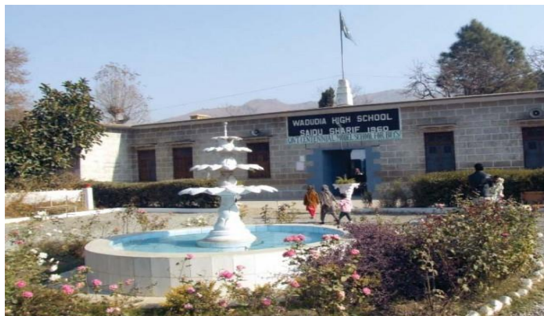
Fig 1: Front view of Waduadia School old building
