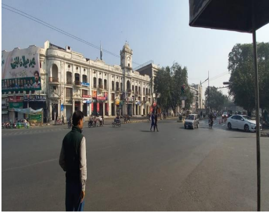
Figure 1 Regal Center Mall Road Lahore
