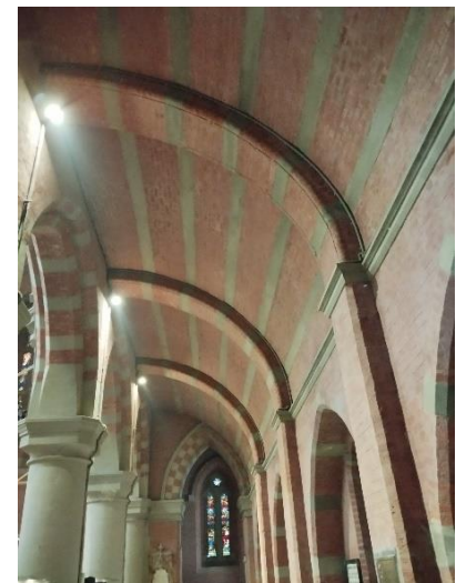
Fig.9 Internal buttresses
