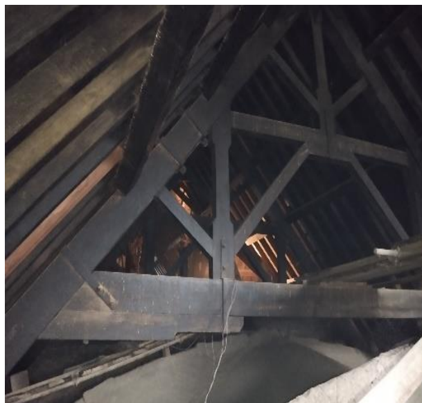
Fig. 5 Wooden roof beams and rafters
