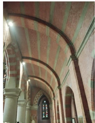
Fig.9 Internal buttresses
