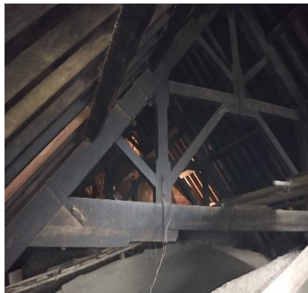
Fig. 5 Wooden roof beams and rafters
