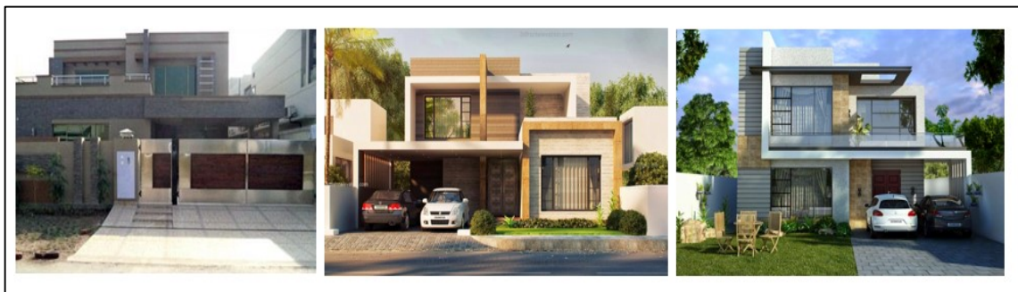
Figure 9 Brick-Concrete Construction of Punjab
