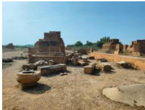
Fig. 2 Damages and deterioration features
